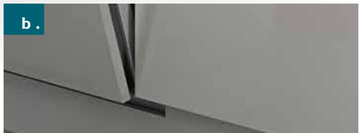
In order to accommodate the swing of the frame, the plinth below the dishwasher requires to be notched.
