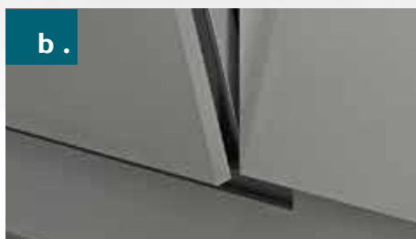
In order to accommodate the swing of the frame, the plinth below the dishwasher requires to be notched.
