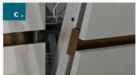
On recessed rail applications, it is recommended that the mid rail end caps are used to conceal the profile edge, resulting in a quality installation.
